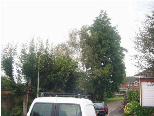
GI looking up Parker Close showing poorly reduced trees in the foreground
